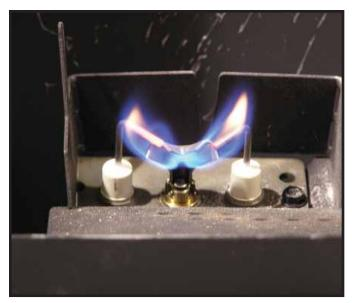
Figure 3.1 IPI Pilot Flame Patterns
